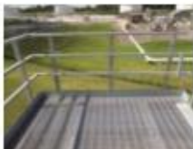
RAILINGS AND DECKING
